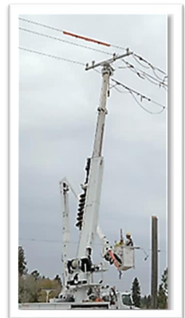
Figure 13. Grid Hardening Work
