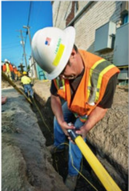
Aldyl A Natural Gas Pipe Replacement
