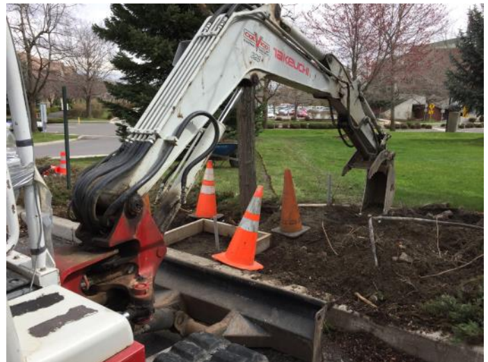
AC level 2 EVSE site construction in partnership with WSU (Riverpoint Campus, 2017)
