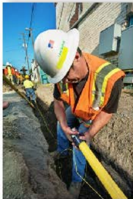
Aldyl A Natural Gas Pipe Replacement
