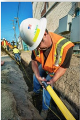
Aldyl A Natural Gas Pipe Replacement
