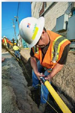
Aldyl A Natural Gas Pipe Replacement
