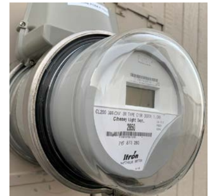
Avista Edge-patented meter collar
