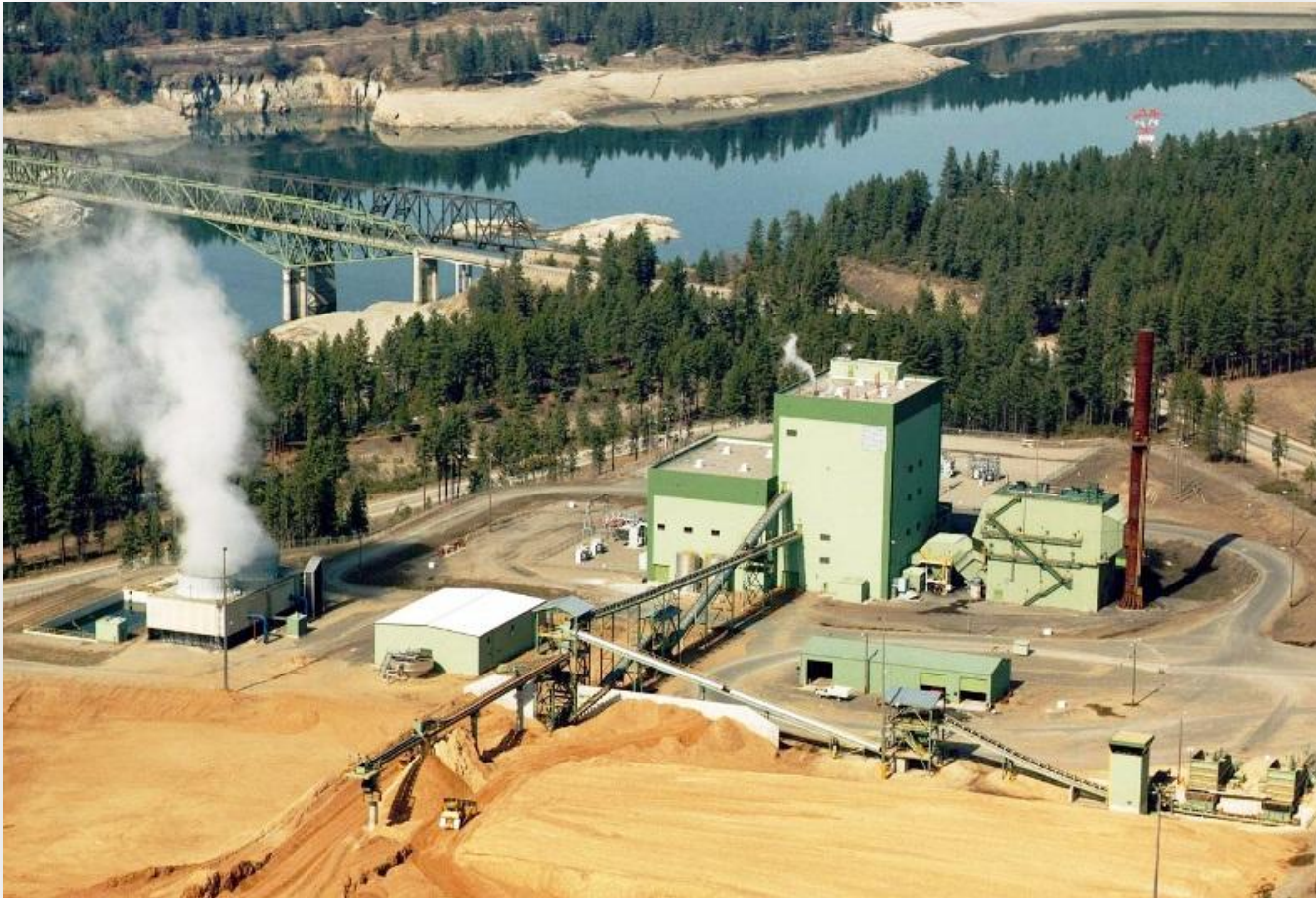
Kettle Falls Generating Station
