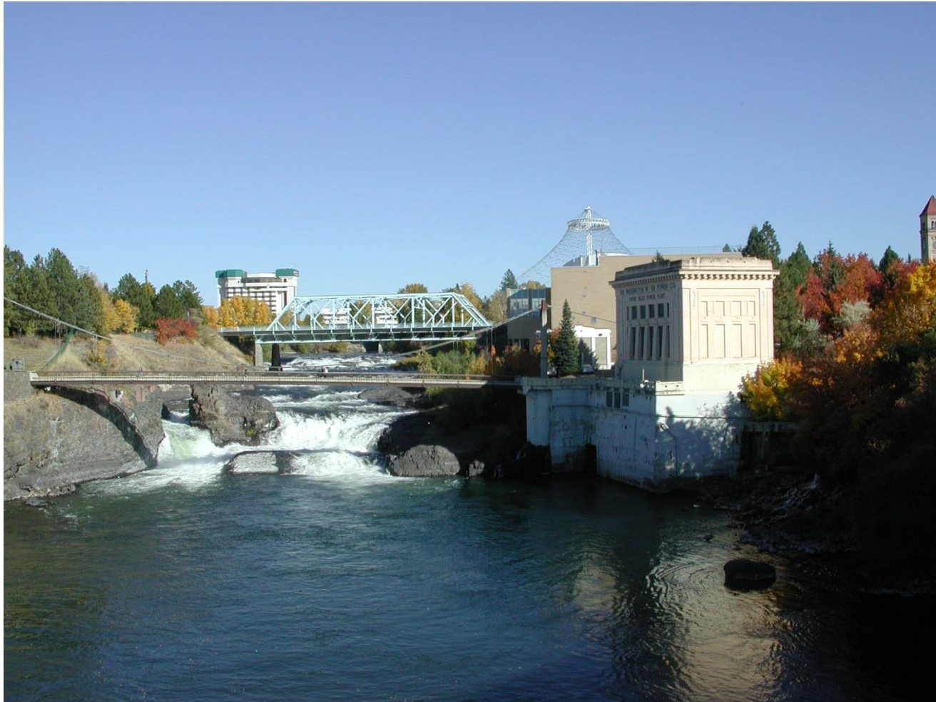
Upper Falls Power Plant Spokane, Wash.
