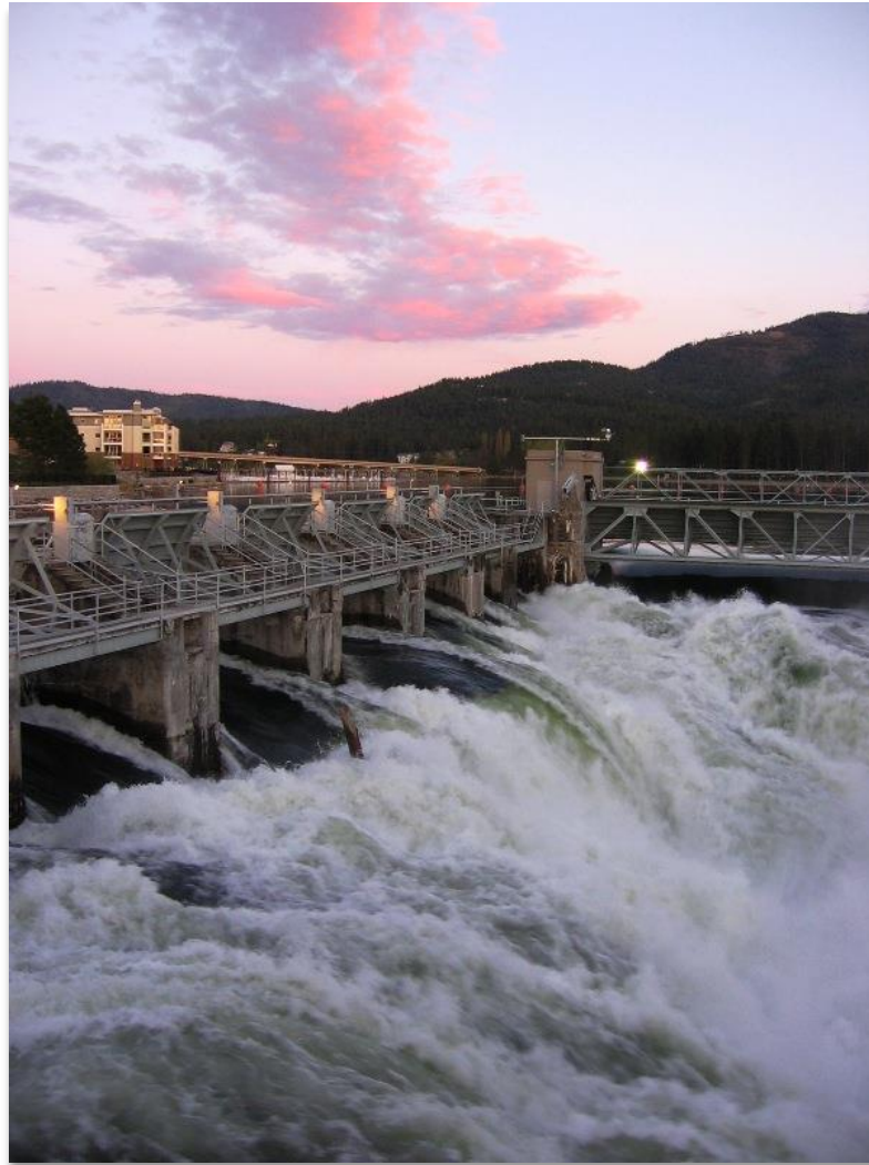
Post Falls Dam Post Falls, Idaho
